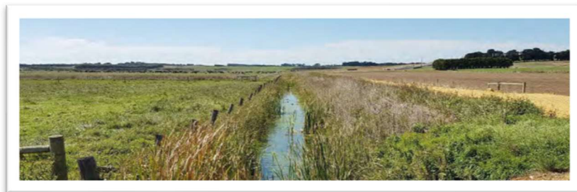
Figure 1: Nullawarre main drain upstream of Skuses Road Bridge. Credit: Glenelg Hopkins CMA
