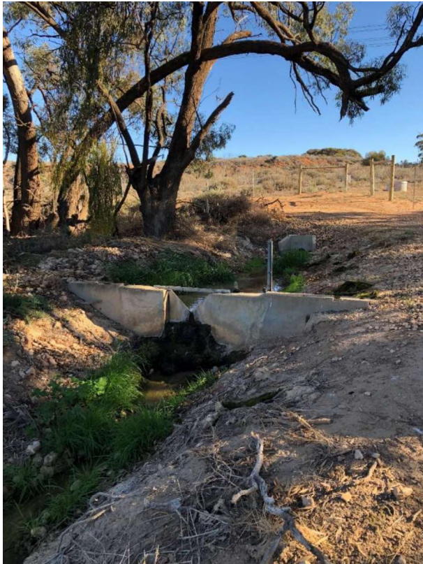
Figure 7 – 414714 Red Cliffs Drain @ Stewarts Road
