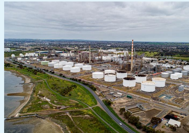
Image 1. Geelong Energy Hub. Credit Viva Energy Australia
