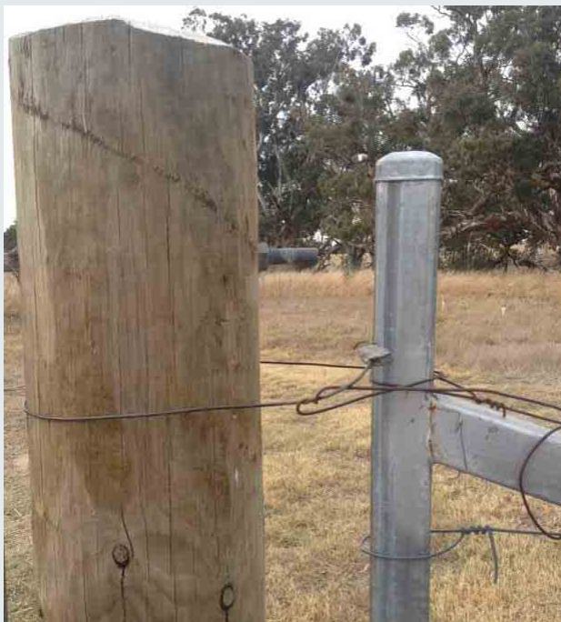
Figure 7.7 – The wire holding the top of the drop-down stay is designed to let go under flood force
