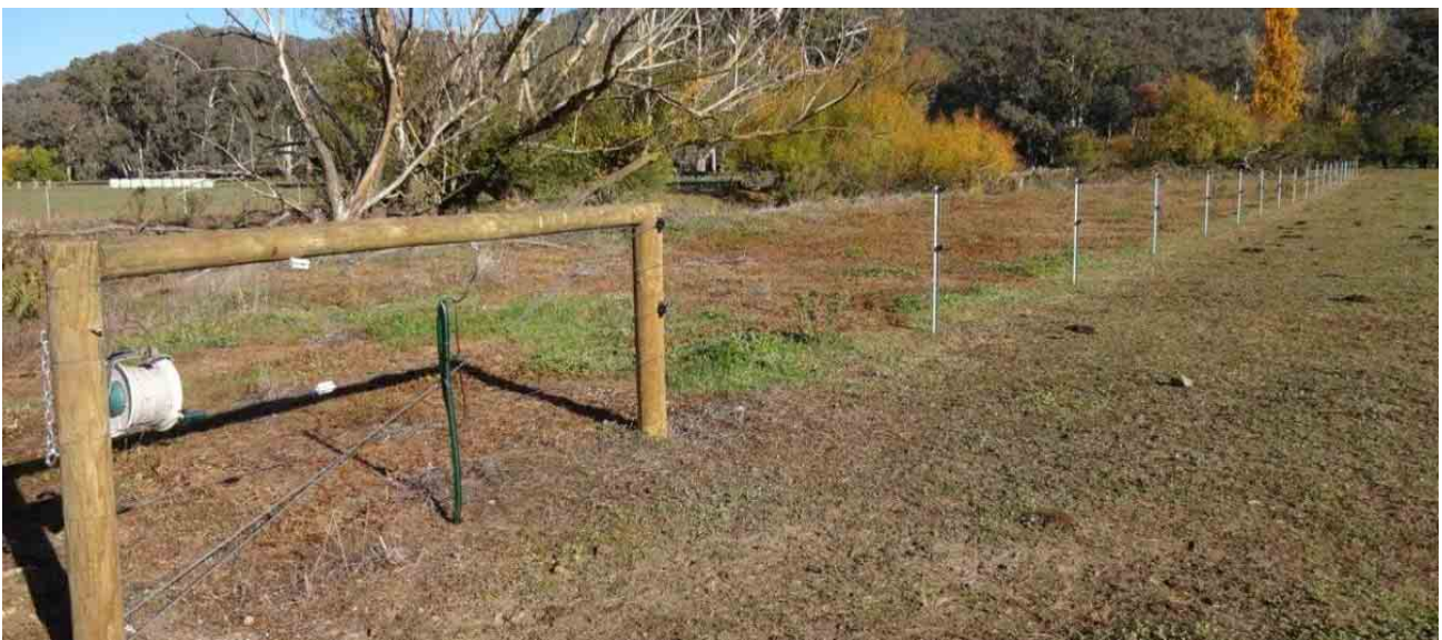
Figure 7.11 – Full-length sacrificial fence
