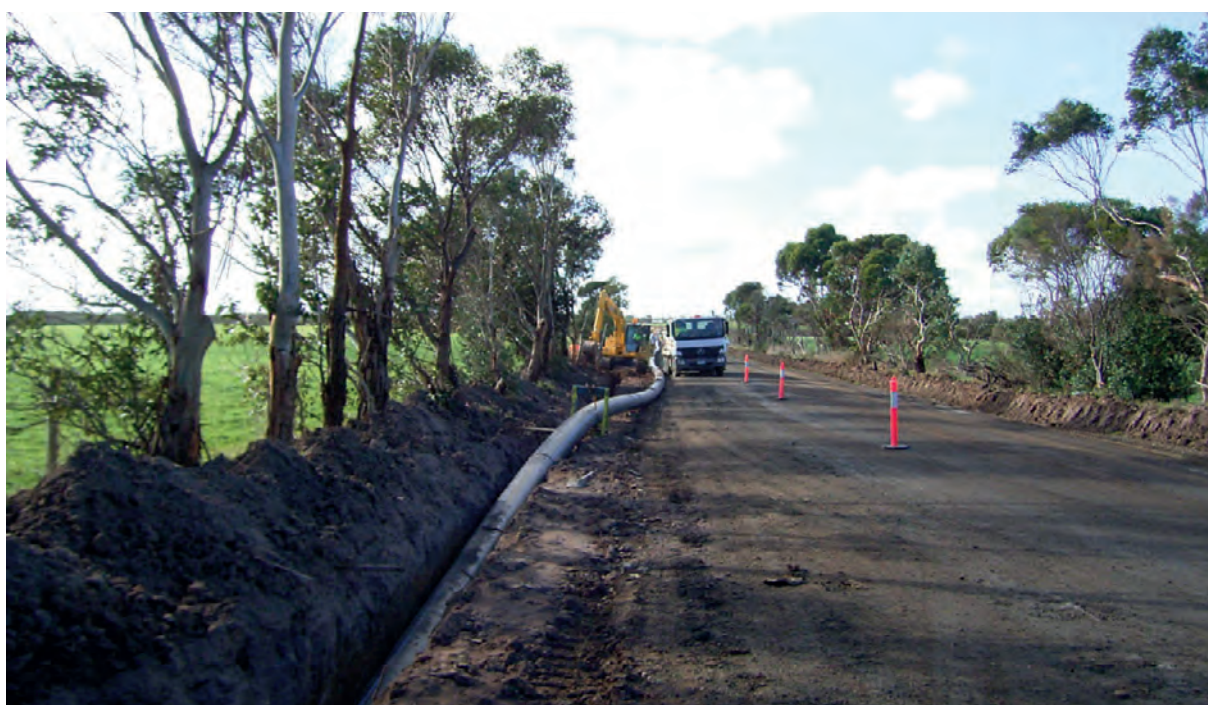
Pipe laying project, SGW
