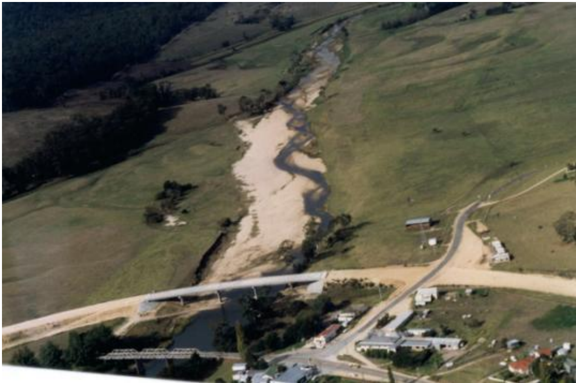
Figure 17. Genoa River following major flooding in 1985 (Photos courtesy of EGCMA)
