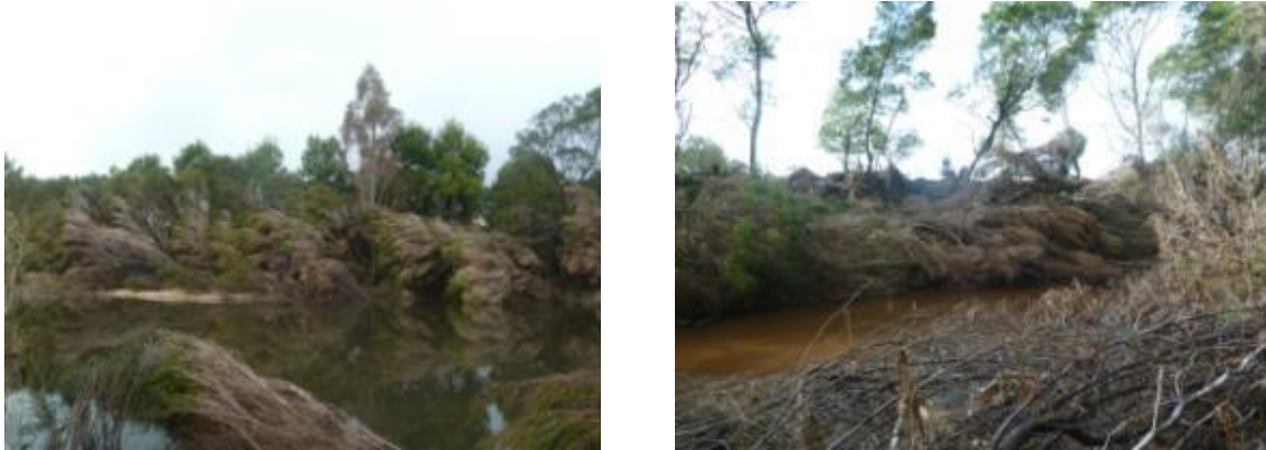
Figure 20. Photos of flood damaged trees on the left and right banks. The force of the floodwater was enough to flatten the 4-5 m trees however the vegetation was still able to protect the banks from scour
