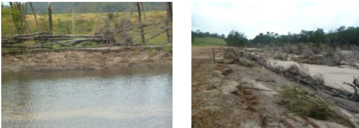
Figure 21. Banks that exhibited localised erosion were limited to areas cleared for stock watering access.
