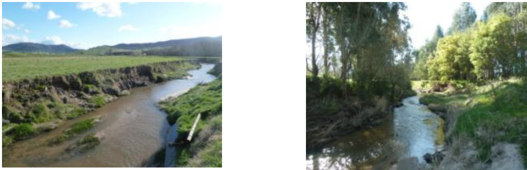
Figure 3. Paired site assessment for Barwidgee Creek, north east Victoria (the site with bare banks (left) experienced widespread erosion while the revegetated site (right) incurred only minor channel change in the same flood event
