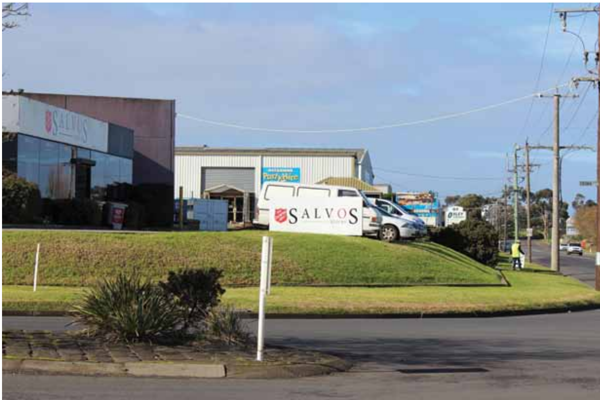
Floor levels constructed higher than the 1% AEP flood level. Source: Simone Wilkinson, DELWP
