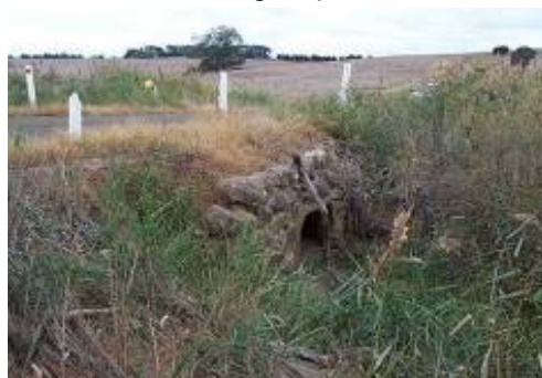
Modified culvert arrangement at road crossing, Unnamed Creek near Coleraine
