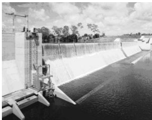
Walla Weir on the Burnett River near Bundaberg, QLD.
