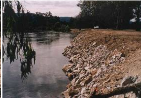
Rock beaching covering battered bank, Murray River (Photo courtesy Tony Crawford, DIPNR)
