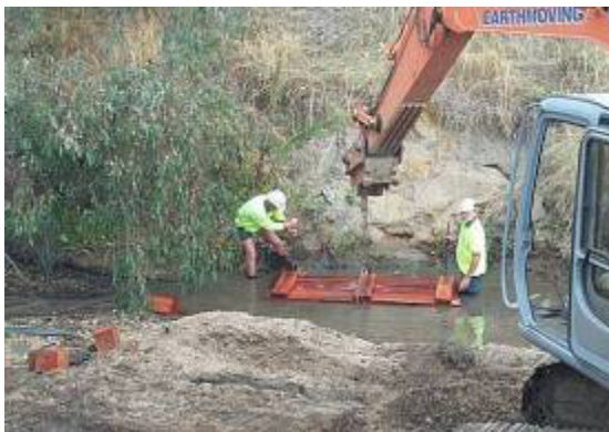
LUNKERS installation upper Goulburn River (Photo courtesy of Goulburn Broken CMA)
