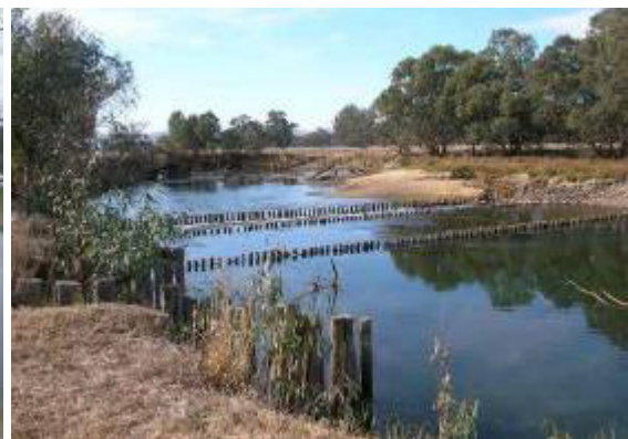
Pile fields combined with bed seeding, Dights Ck, River Murray, NSW
