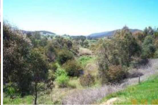
Rock chute in Barwidgee Creek (Ovens River Catchment) 2002
