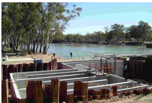
Vertical slot fishway construction at Torrumbarry Weir, River Murray
