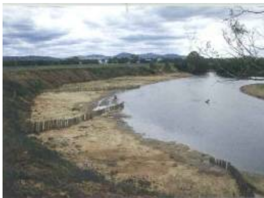
Pile fields, Wodonga Creek, north east Victoria
