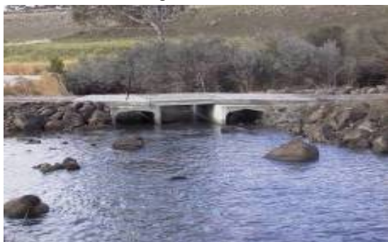
Modified culvert arrangement at road crossing, Barwon River near Deans Marsh
