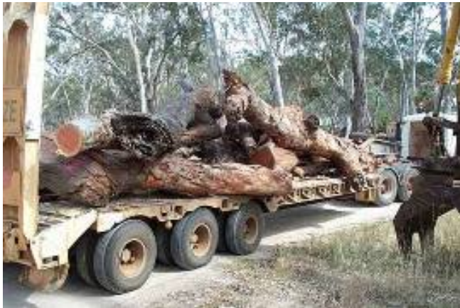
Large wood for installation, Glenelg River at Harrow
