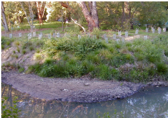
Revegetation works at Gardiners Creek (Photo courtesy of Earth Tech)
