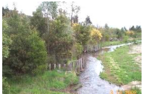
Black Range Creek, north east Victoria, 6 years following works alignment training works
