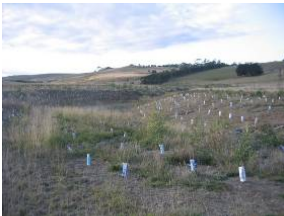
Battered banks combined with a grass chute and revegetation, Retreat Creek, western Victoria
