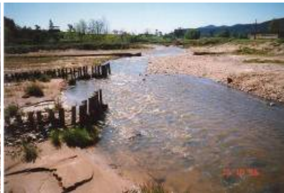
Pile field Black Range Creek, north east Victoria
