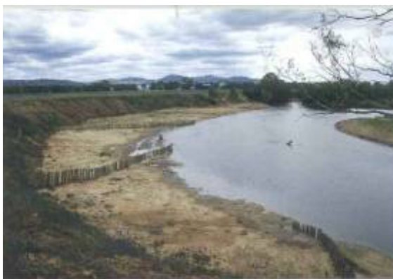
Pile fields for alignment training, Wodonga Ck, north east Victoria
