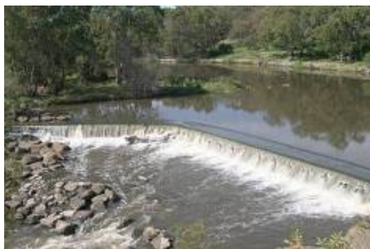
Rock fishway at Dights Falls, Yarra River, Melbourne (Source: http://en.wikipedia.org/wiki/ )
