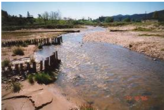
Black Range Creek, north east Victoria, immediately following pie field based alignment training to manage sediment loads and channel instabilities
