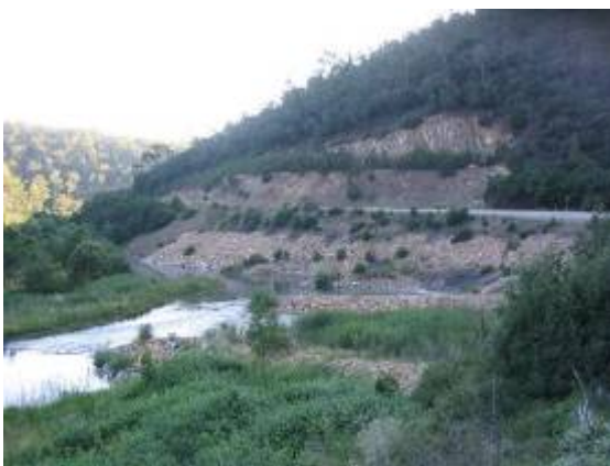
Rock groynes, Tambo River, East Gippsland
