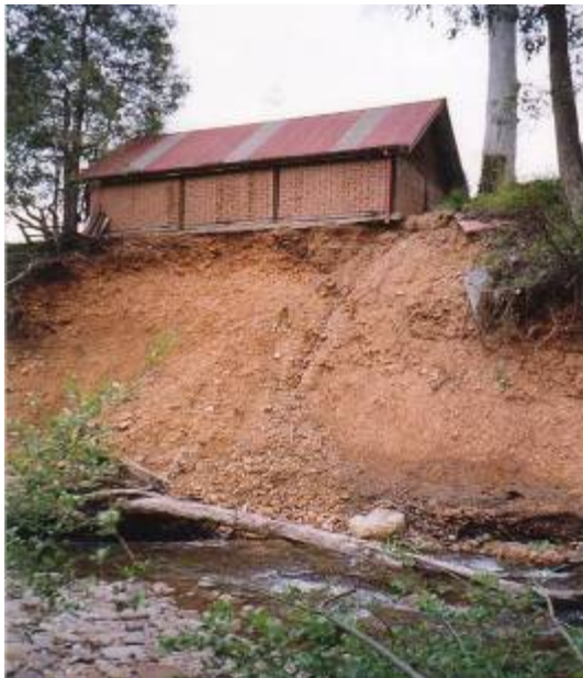
Stream bank erosion, Ovens River catchment
