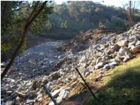
Decommissioning of Honeysuckle Reservoir (Image courtesy of Earth Tech)
