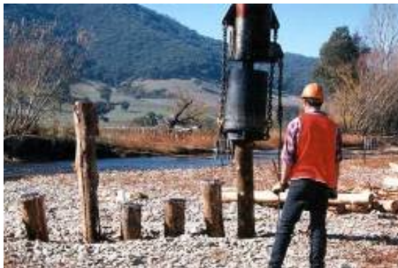
Pile field installation Ovens River, north east Victoria
