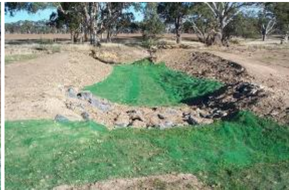
Grass chute construction near Stawell catchment
