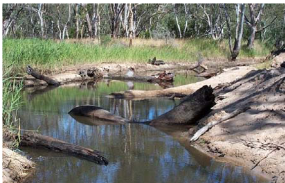
Large wood installation, Glenelg River at Harrow
