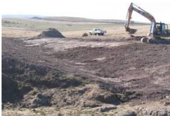
Grass chute construction retreat Creek, near Deans Marsh
