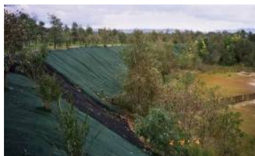
Wodonga Creek following bank battering
