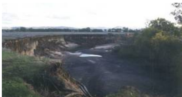
Wodonga Creek prior to bank battering
