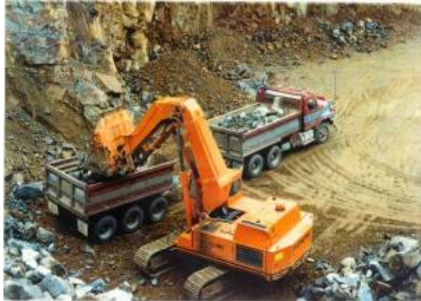
Everton Quarry north east Victoria
