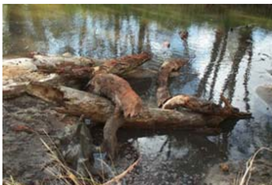
Engineered log jam on Glenelg River at Harrow
