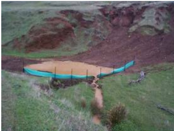
Instream sediment trap, Adelaide Hills, South Australia
