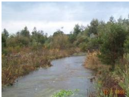
Pile and rail alignment training (in background) and revegetation, Black Range Creek, north east Victoria
