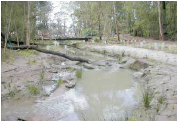
Revegetation works Blackburn Creek, Blackburn (Image courtesy of Earth Tech)
