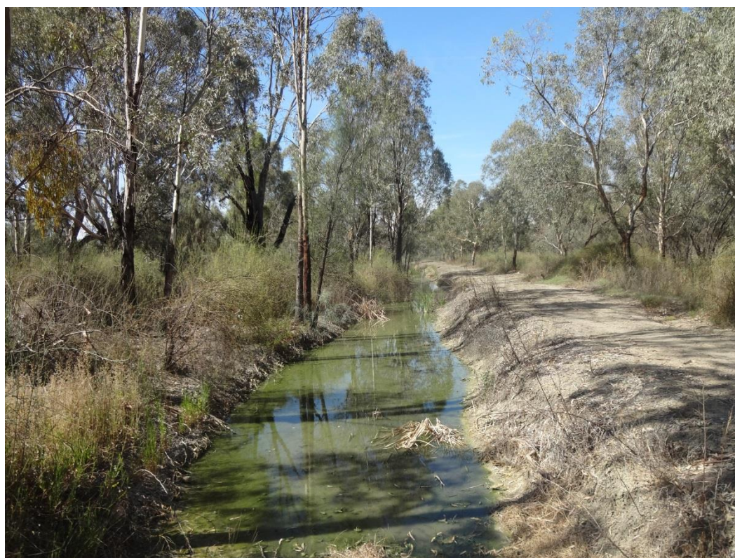
Figure 14 - Irrigation drainage channel running through wetland #7428653680, showing algae, weed control and excavation works near drain confluence with the Murray River.
