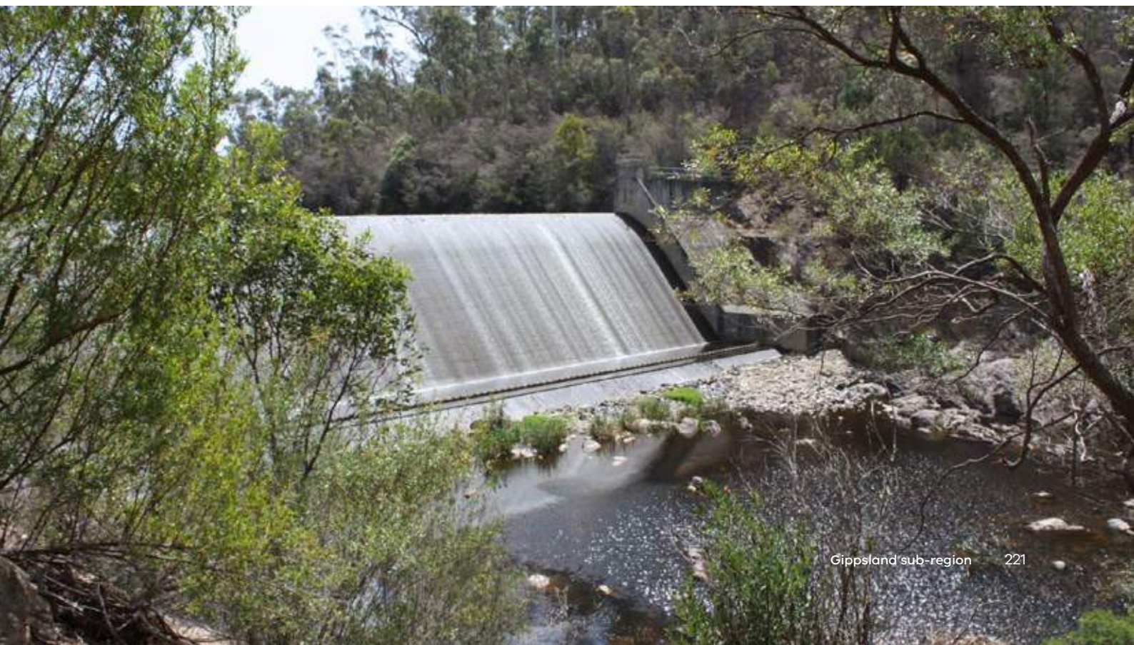
Image: Nicholson River Dam wall
