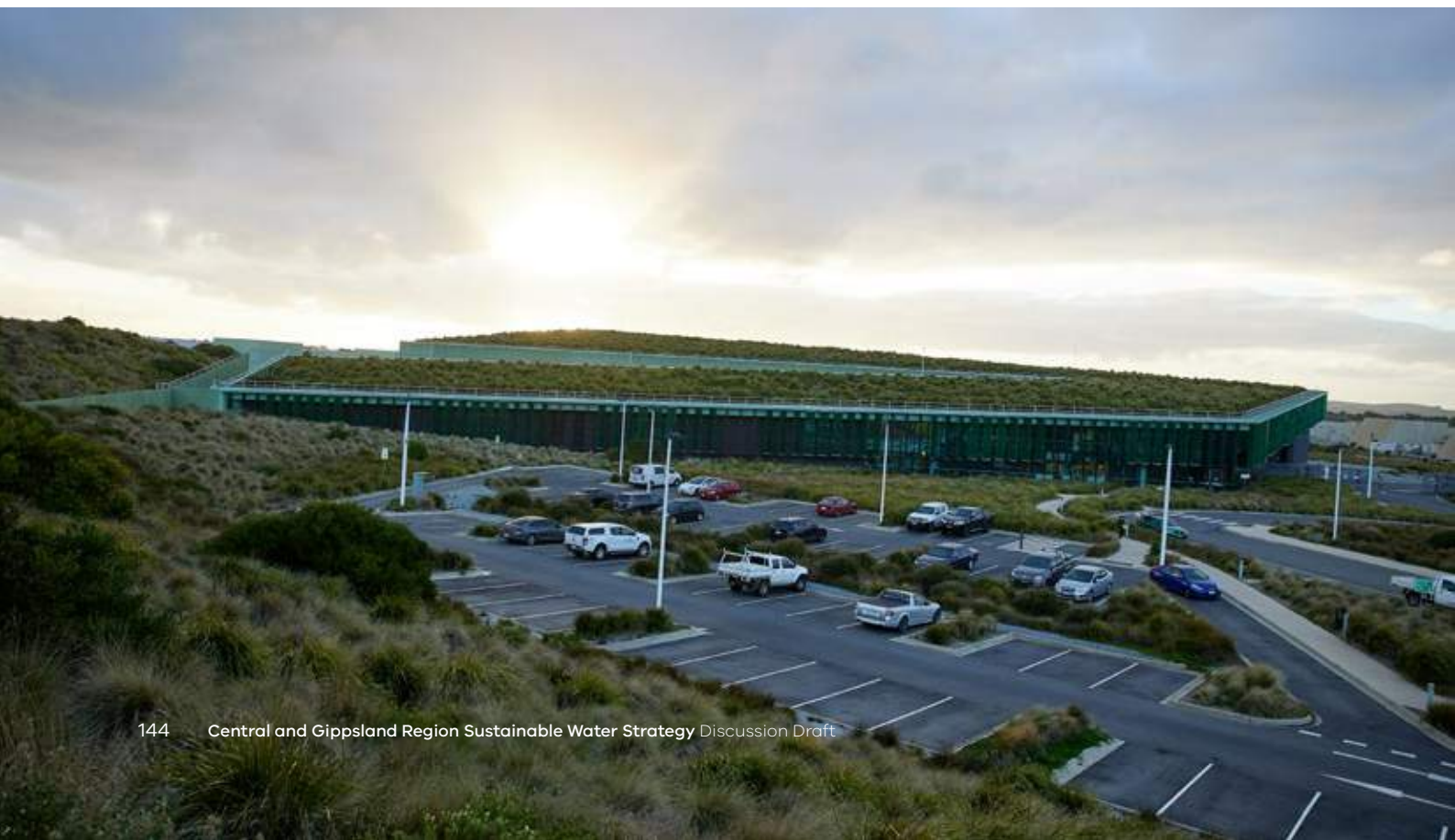
Image: Victorian Desalination Project, Wonthaggi, Bunurong Country
