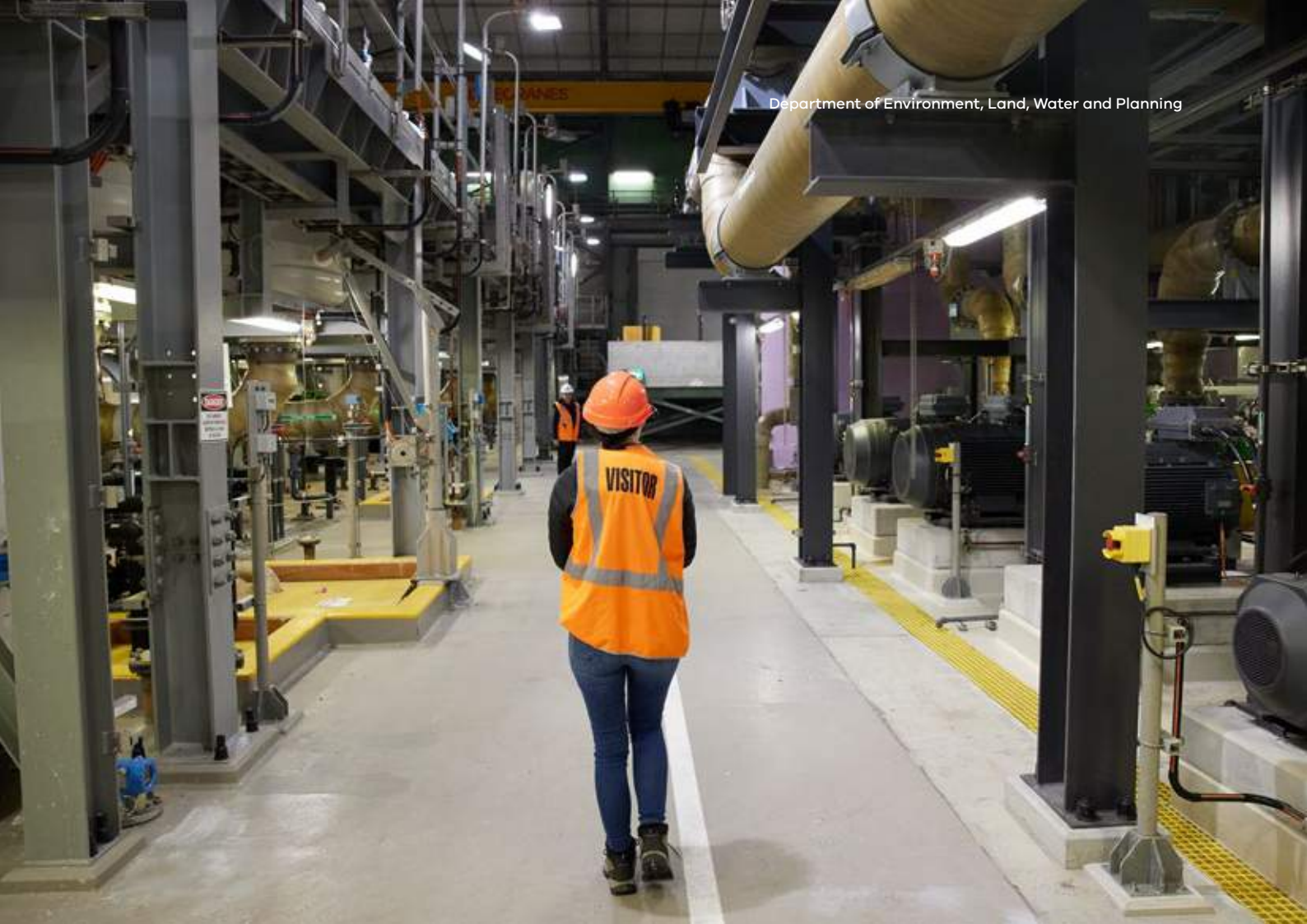
Image: Worker at the Victorian Desalination Project, Wonthaggi, Bunurong Country
