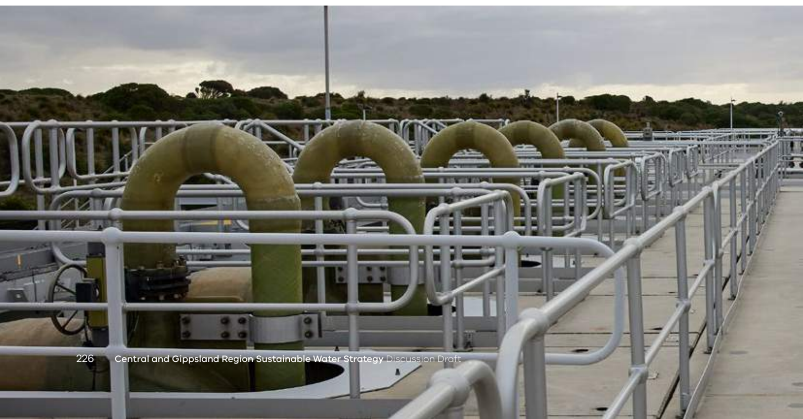
Image: Victorian Desalination Project, Wonthaggi, Bunurong Country
