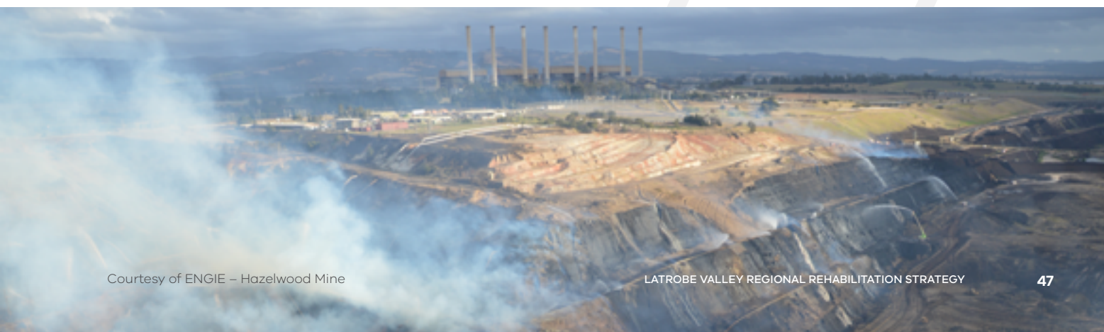
Figure 6: Burning batters during the Hazelwood mine fire
