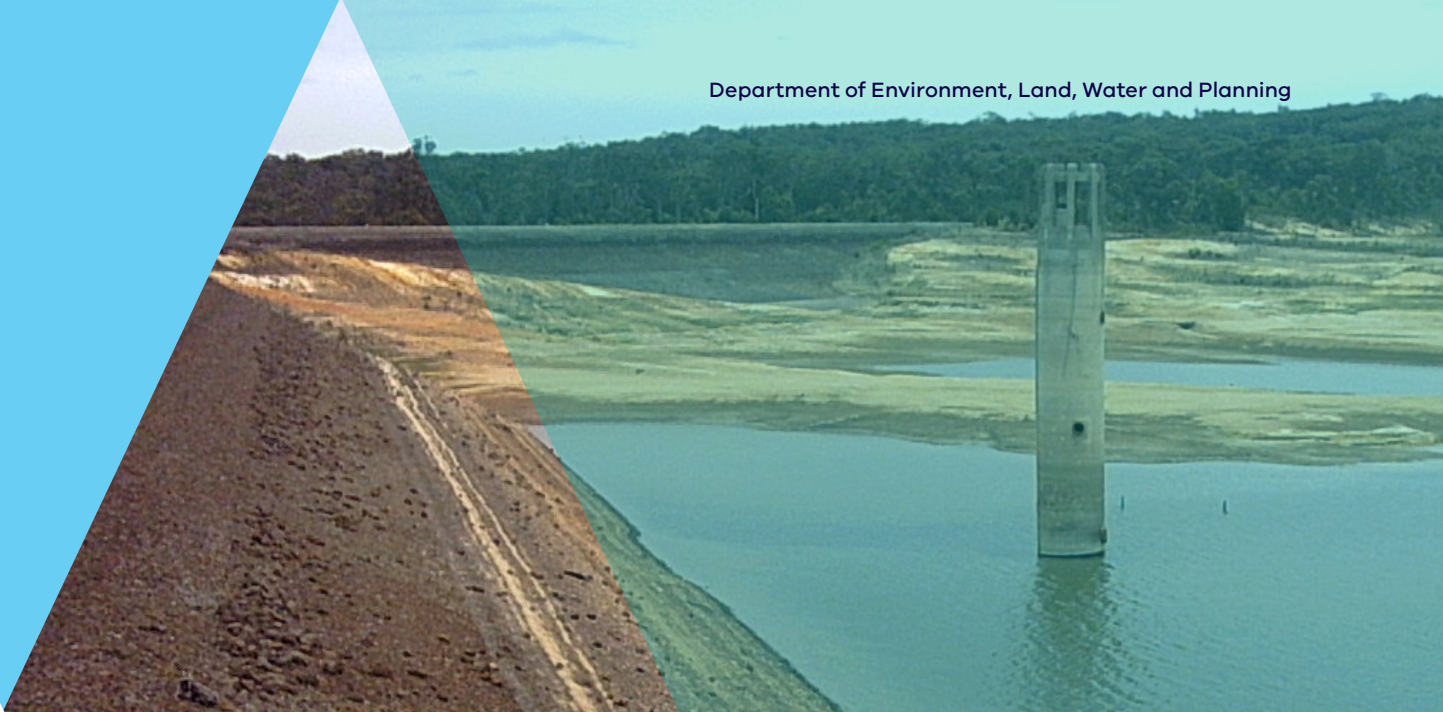
White Swan Reservoir, a critical supply for the Ballarat system, near its lowest level — 946 ML, or 6.7% of capacity — in April 2008. The total Ballarat system bottomed out at 4,693 ML (7.2%) — about three months' supply — in May 2008. Image: Central Highlands Water
