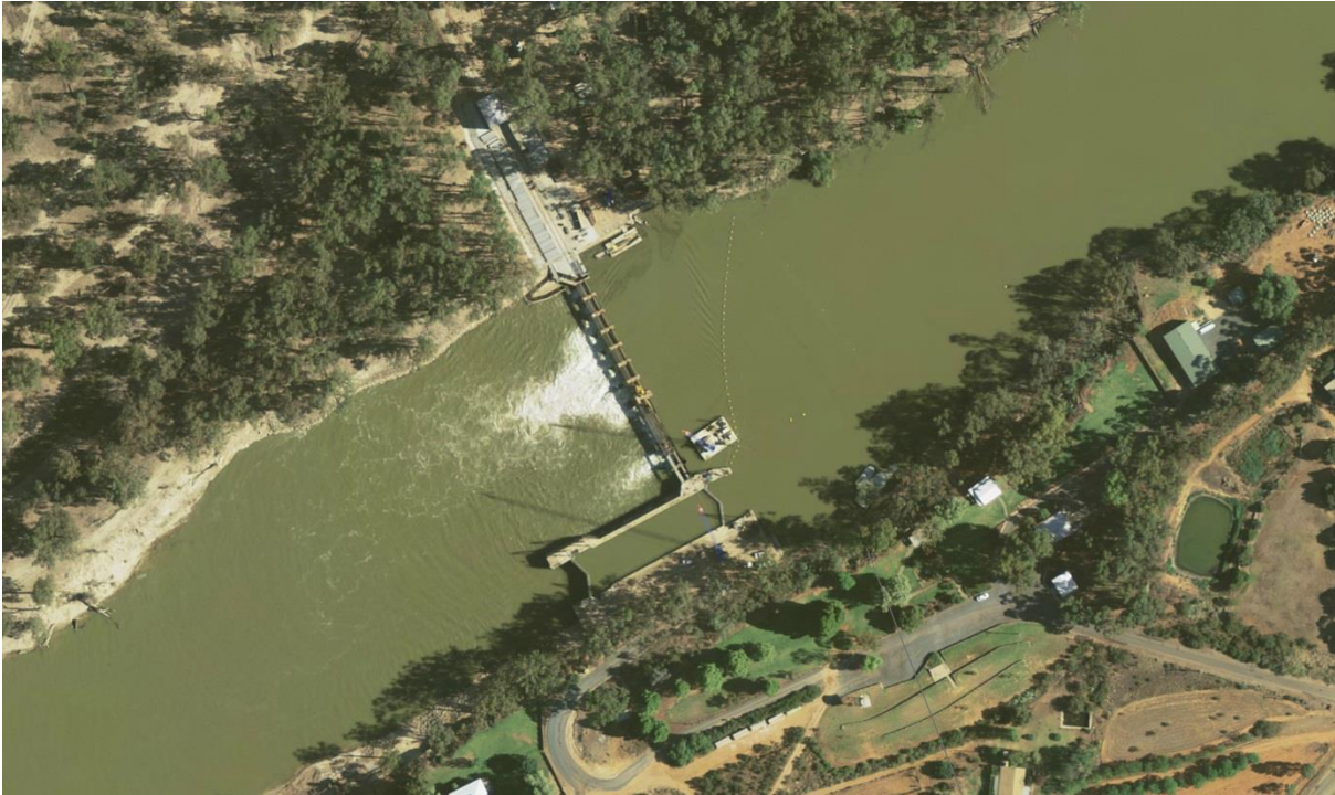
Figure 22. Lock & Weir 15 showing the lock on the South (Left) bank. The fishway is on the North (Right) bank located between the lock chamber and the weir section.
