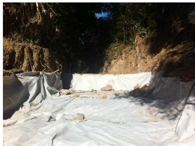
Figure 80. Application of geotextiles (Source: S. Cleven).
