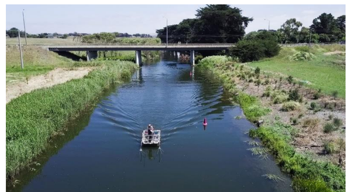
Merri River before and after riparian improvement works. Image courtesy Glenelg Hopkins CMA.
