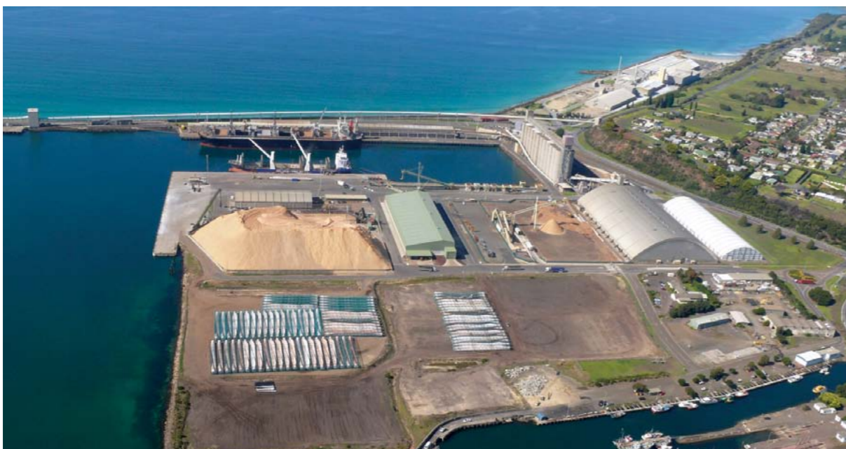
Port of Portland - aerial view
