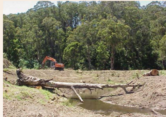
Gellibrand River project site during restoration (December 2002)
