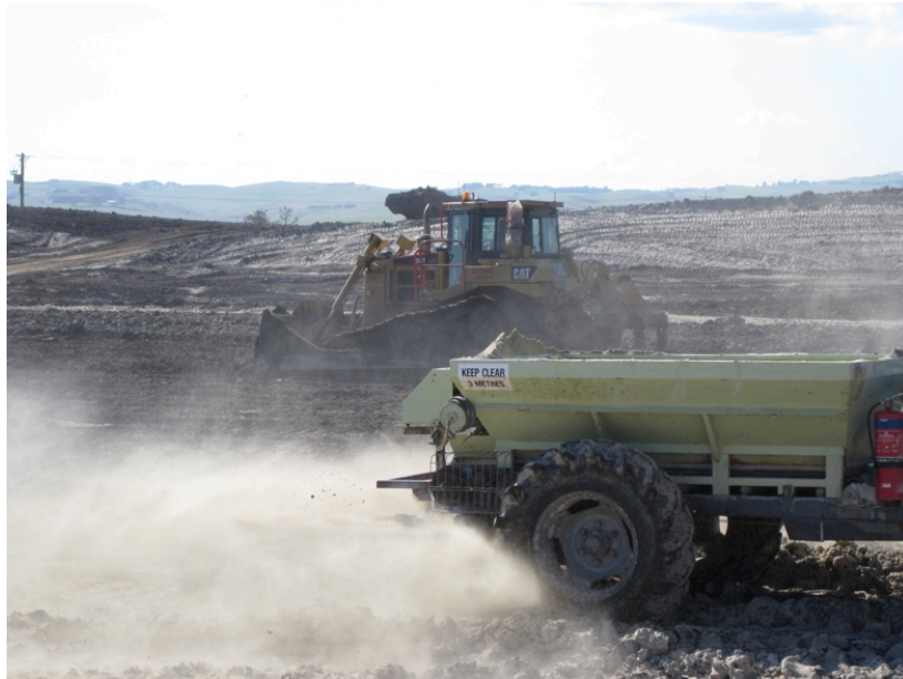
Figure 6. Acid sulphate soils treatment, May 2011
