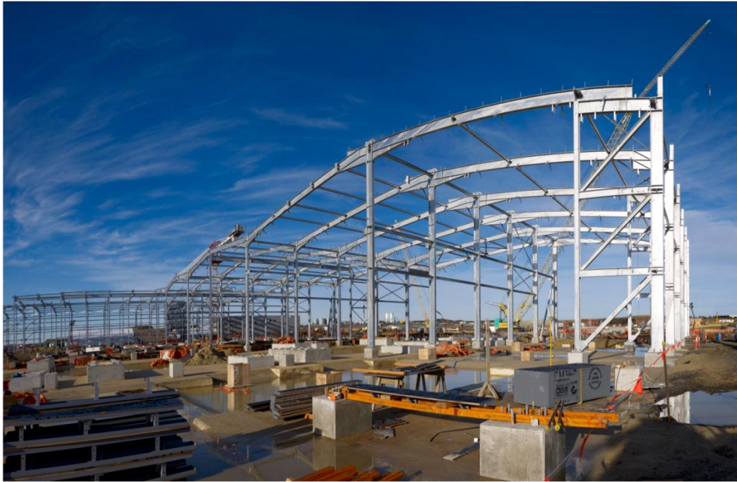
Figure 3. Reverse Osmosis Building construction works, June 2010
