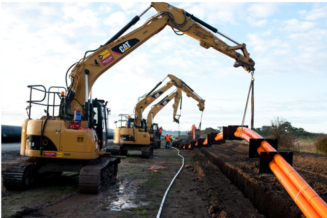
Figure 4. Laying the power cable conduit.
