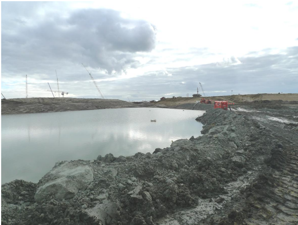
Figure 6. Plant site construction water sediment pond, July 2010
