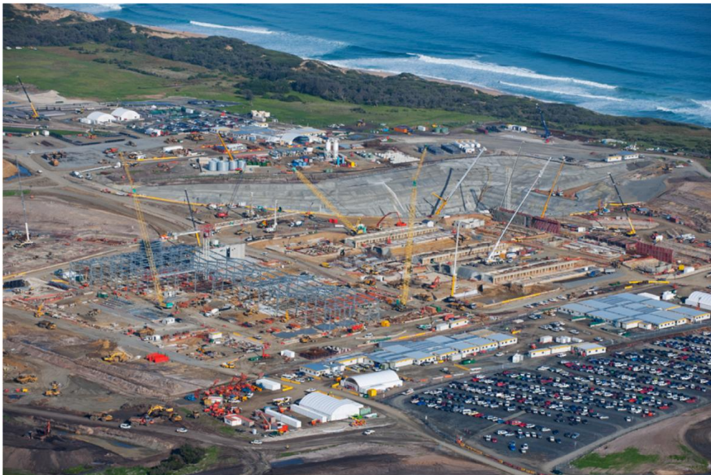
Figure 2. Overview of plant site construction. June 2010
