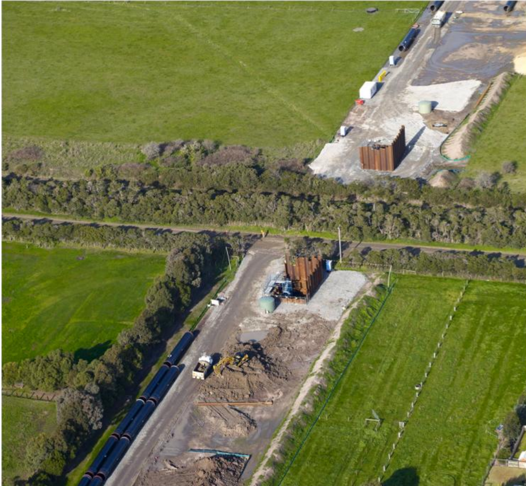
Figure 7. Preparation for a pipe-jack waterway crossing
