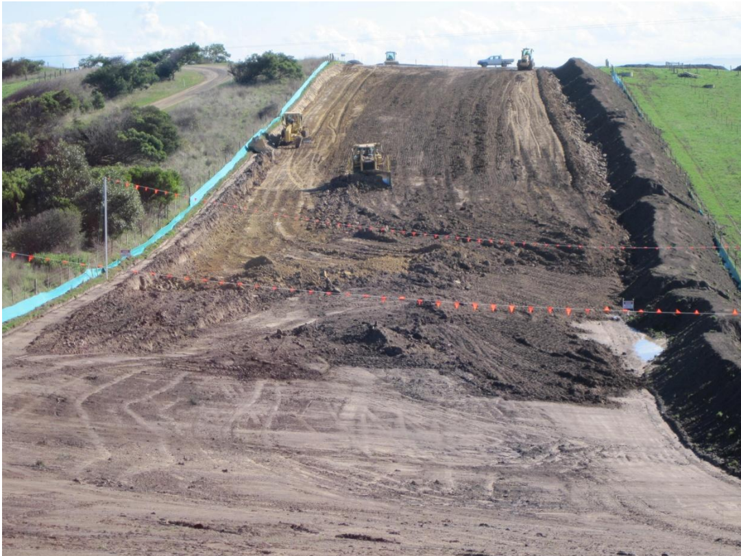
Figure 5. Clearing and grading the Right of Way, June 2010
