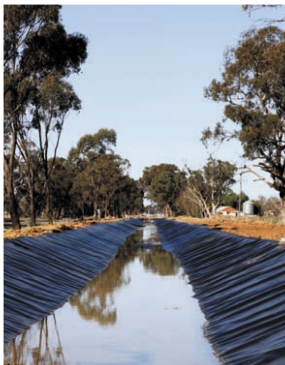
New channel lining, Central Goulburn
