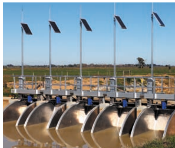
Channel modernisation, Pyramid-Boort
