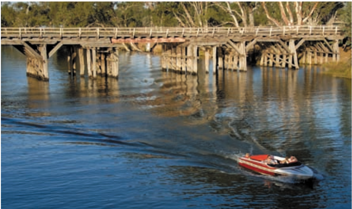
Chinaman's Bridge, Goulburn River
