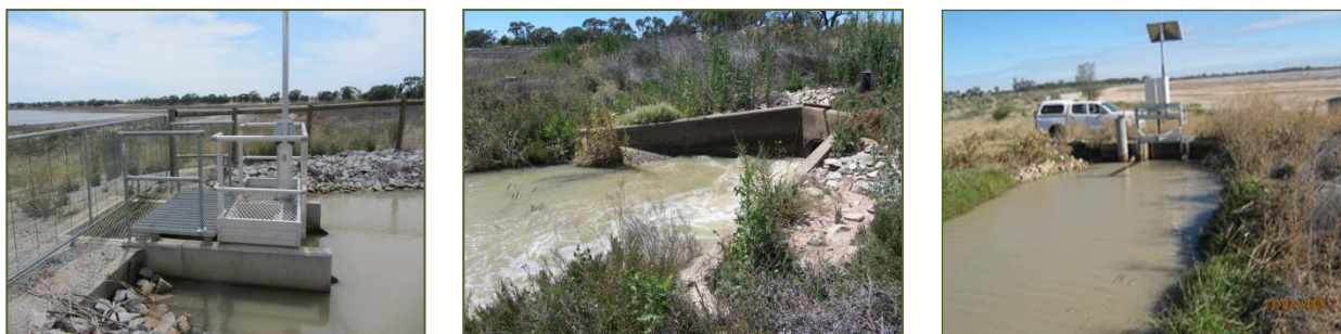
Figure 10: Infrastructure at Lake Elizabeth. Left: 28/2 outfall structure, middle: culvert, right: 28/2 channel
