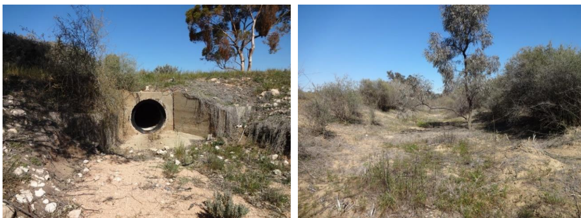
Figure 5 - Culvert under the Murray Valley highway and the spoon drain which allows inundation of Heywood Lake either through flood event or pumping of environmental water
