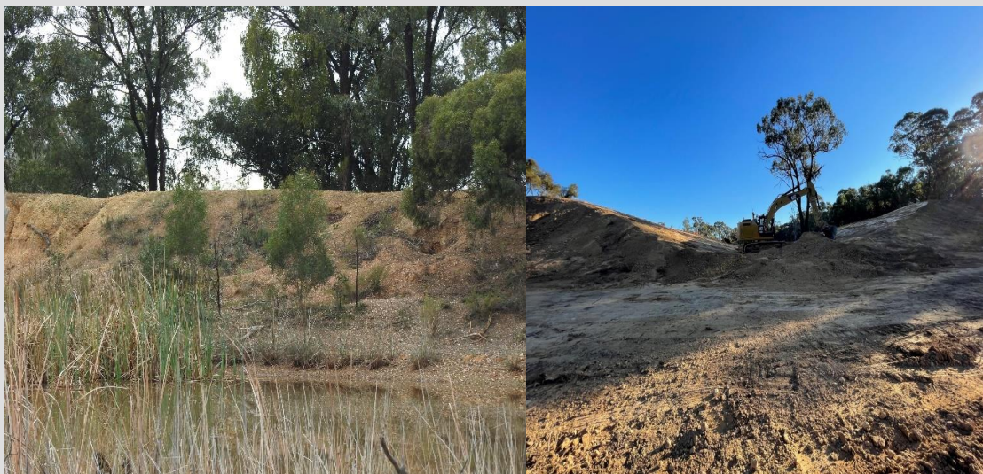
Figure 6. Nine Mile dam wall before (left) and during (right) decommissioning works
