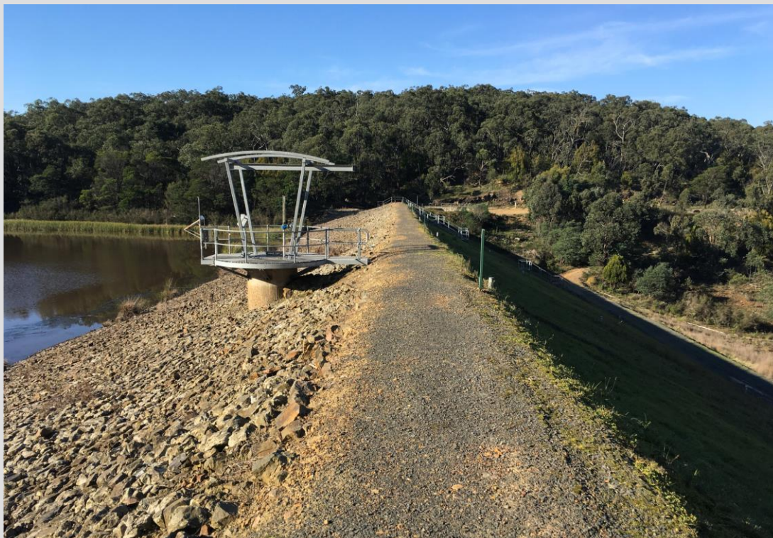
Figure 8: Beaconsfield dam wall view from right hand side of crest.
