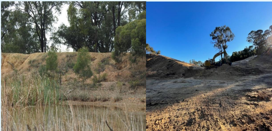
Figure 8: Nine Mile dam wall before (left) and during (right) decommissioning works
