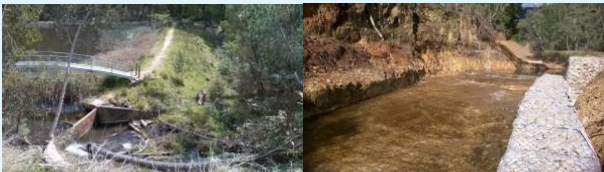
Figure 7: Bakers Gully Lower Reservoir before (left) and after (right) decommissioning
