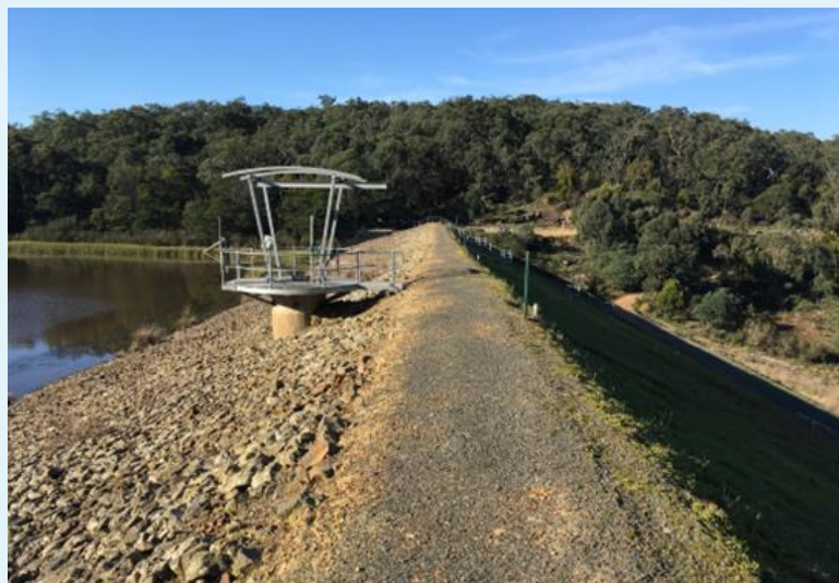
Figure 10: Beaconsfield dam wall view from right hand side of crest
