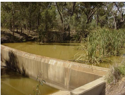
Figure 6. Fixed crest weir historically used to pool water from Lockington Main drain and force it into Richardson's Lagoon. DSE (A. Joyce) 2005.
