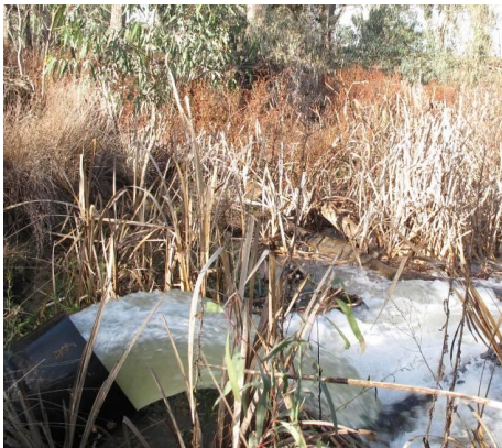
Figure 9. Pipe outfalling to Link Channel before entering wetland proper.
