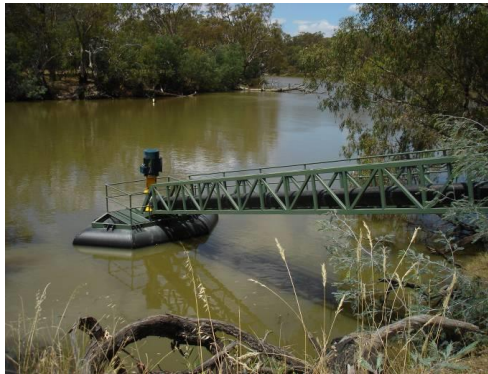
Figure 8. Fixed pontoon pump on Murray River to provide water to Richardson's Lagoon. DSE (A. Joyce)
