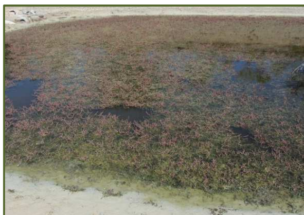
Pond Weed in dam (29 April 2012) at Falla Dam
