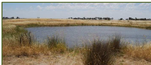
Creswick Dam, December 2013 (K. Howard [ARI] 2014)
