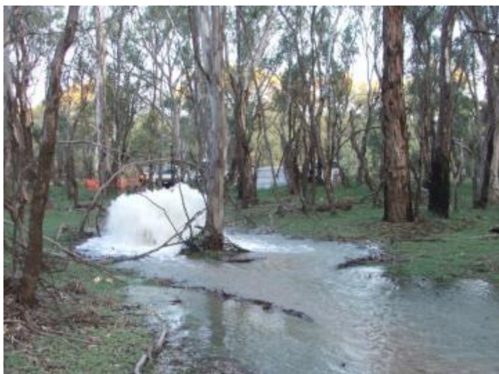
Pumping at Nyah, April 2010
