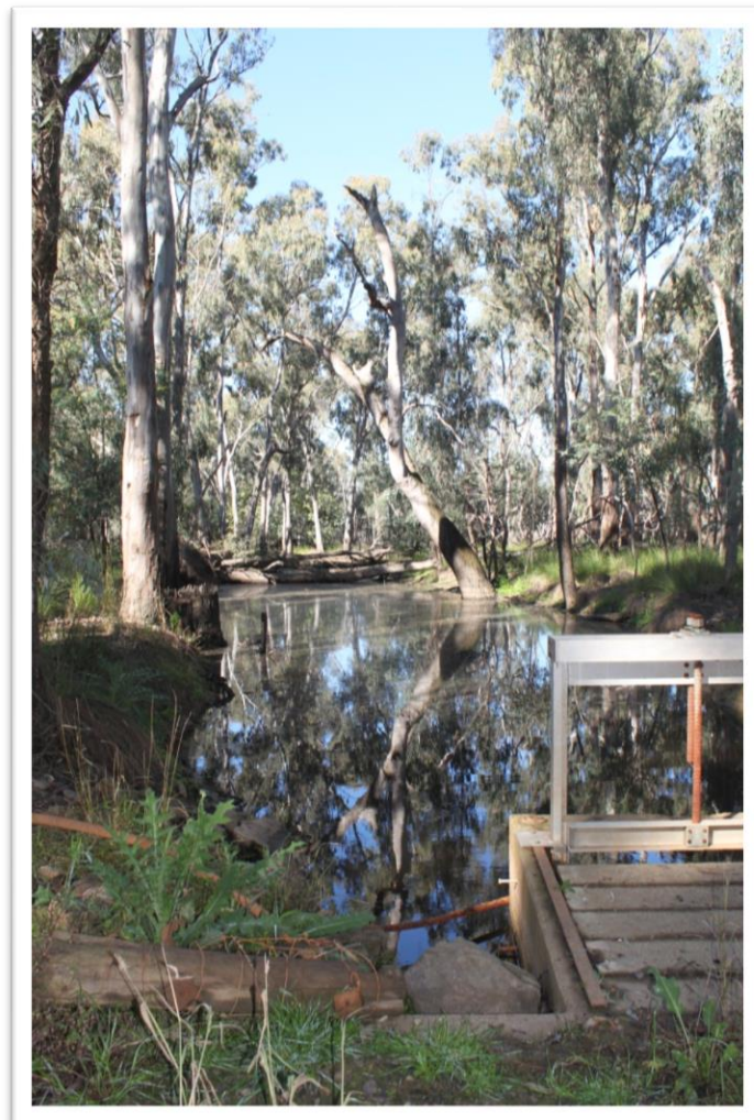
Figure 9: The outlet structure on North Creek at Reedy Swamp, constructed in 1979.
