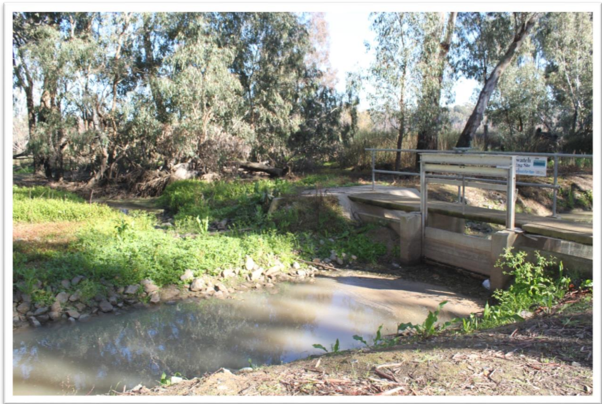
Figure 10: Regulating Structure and overflow sill at Reedy Swamp to allow drainage water in the wetland as required.
