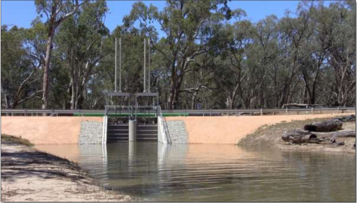
The Messengers environmental regulator, constructed under The Living Murray program during 2012-13
