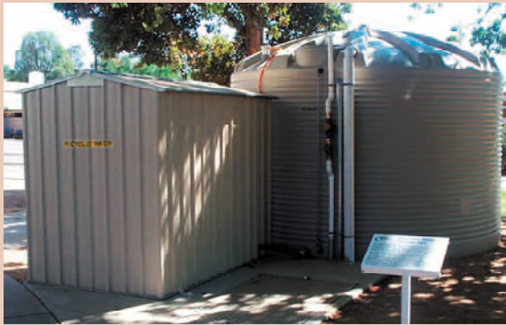
Water conservation and recycling for Bendigo Photographer: Bendigo Health Care Group
