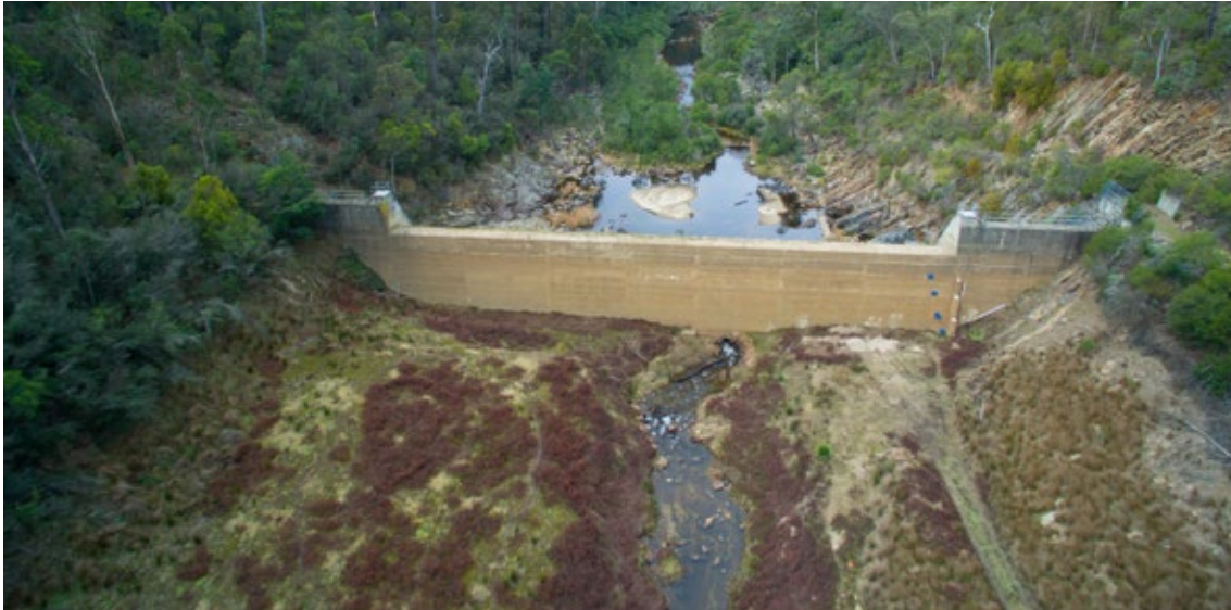
Figure 7: Aerial image of Nicholson Dam facing downstream. Image courtesy of East Gippsland CMA
