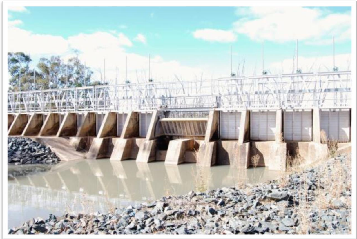
Figure 11: Groves Weir regulator and Wanalta Creek
