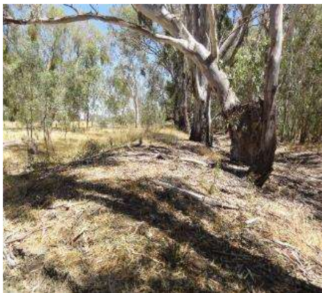
Benwell Forest south levee (Photo: DHI)
