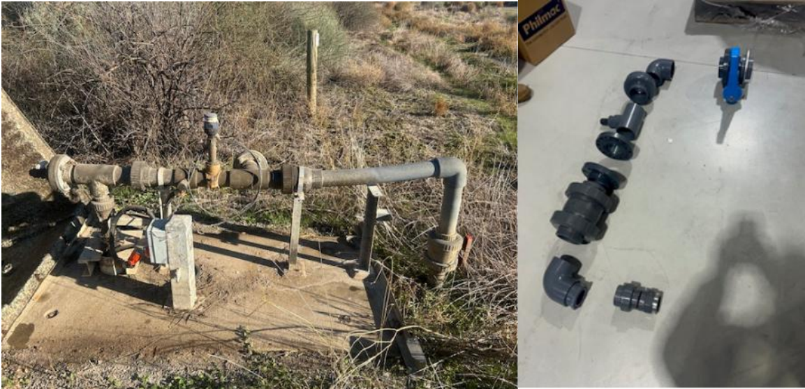
Figure 1: Previous condition of headworks prior to update works. Photo credit: GMW
