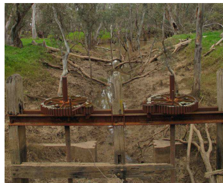
Figure 10. Blackfellows Creek with disused regulating structure, Loddon River in background.
