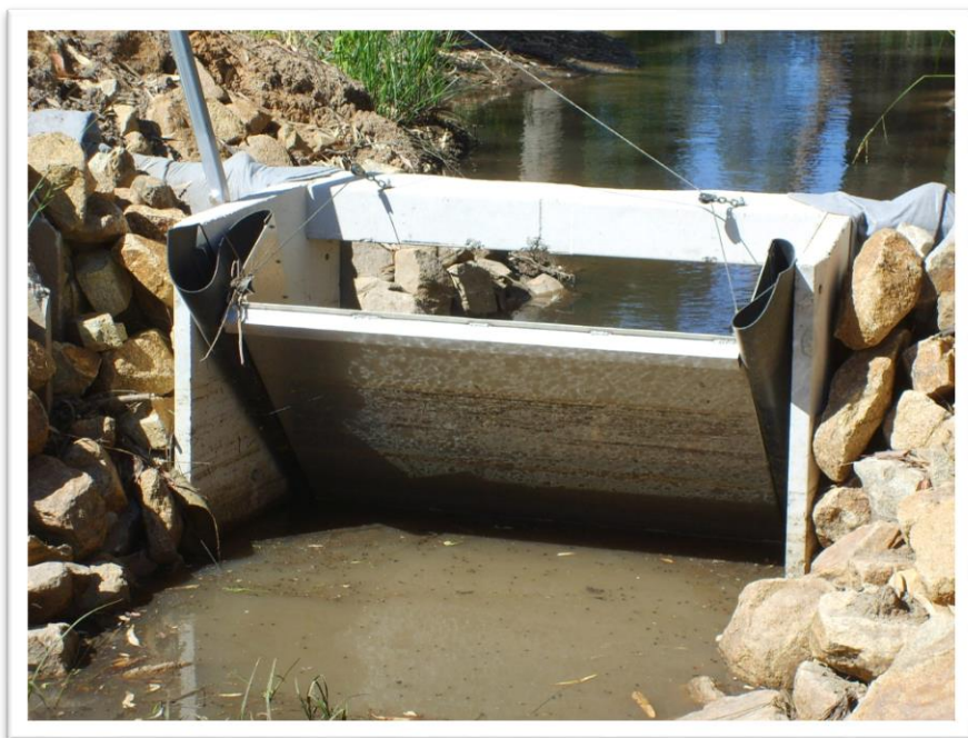
Figure 11: Upgrade of the regulator on the Broken Creek.
