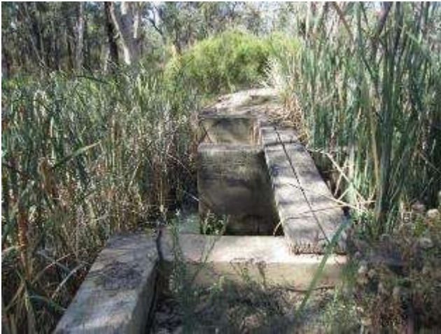
Camerons Creek regulator (Photo: C. Corr)
