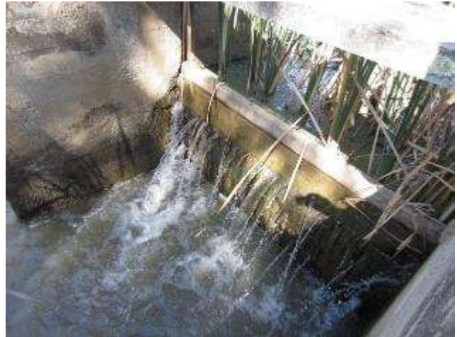
Camerons Creek regulator (Photo: C. Corr)
