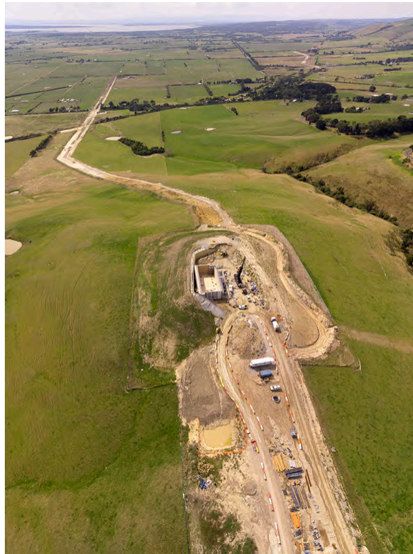
Figure 3. Construction of surge tank, April 2012
