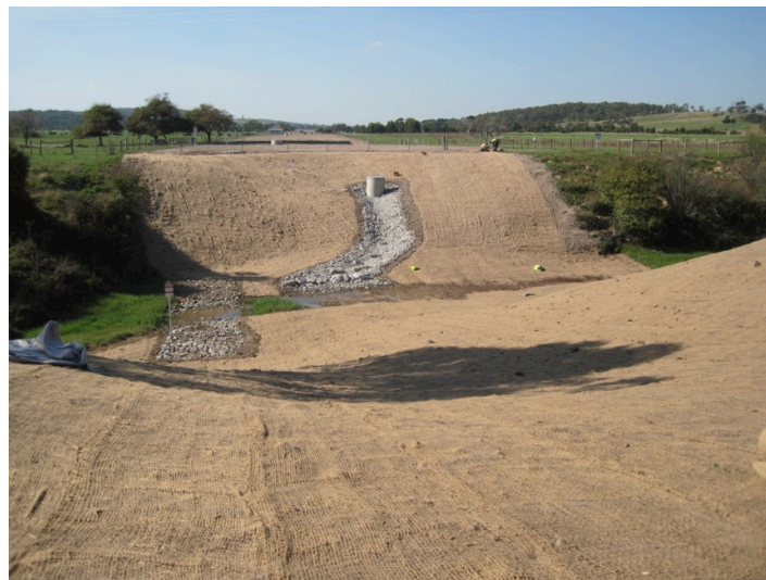
Figure 8. Waterway reinstatement, Utilities alignment, April 2012.
