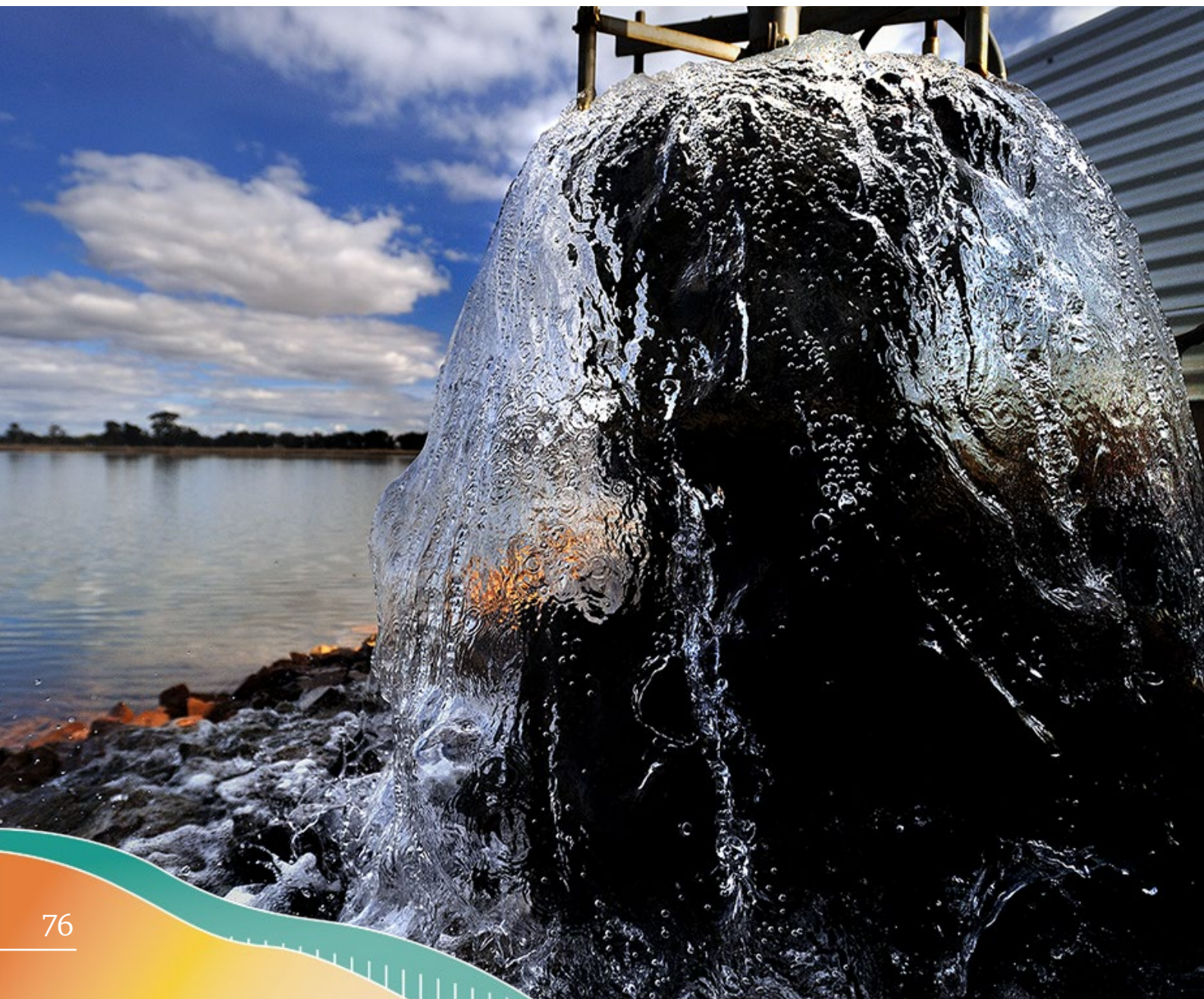
Horsham Water Treatment Works. Photo credit: David Fletcher, GWMWater
