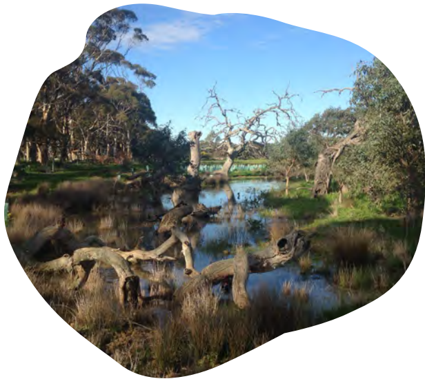
Image: Lollypop Creek water treatment plant
