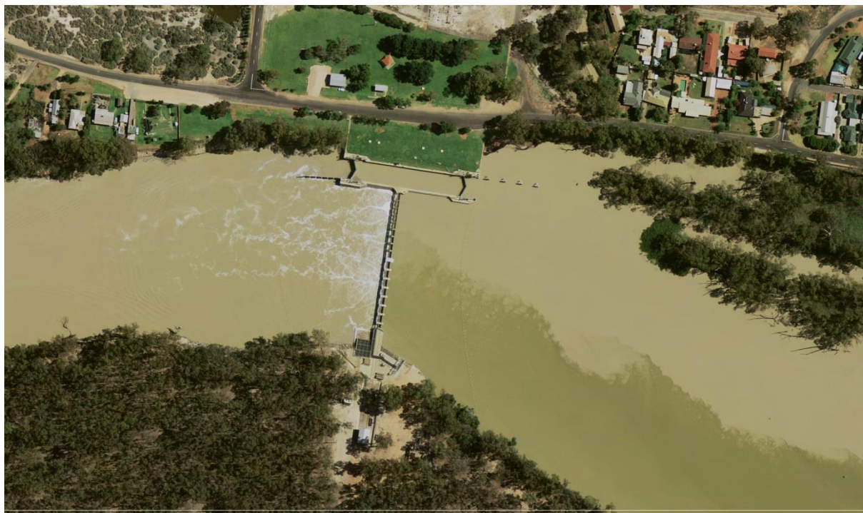
Figure 29. Lock 10 showing the lock on the North (Right) bank. The fishway is on the South (left) bank. (Source: Google Maps)
