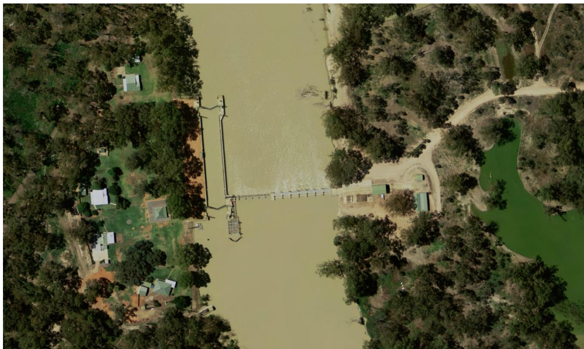
Figure 32. Lock 7 showing the lock on the South (left) bank. The fishway is on the north (right) bank (Source: Google Maps)
