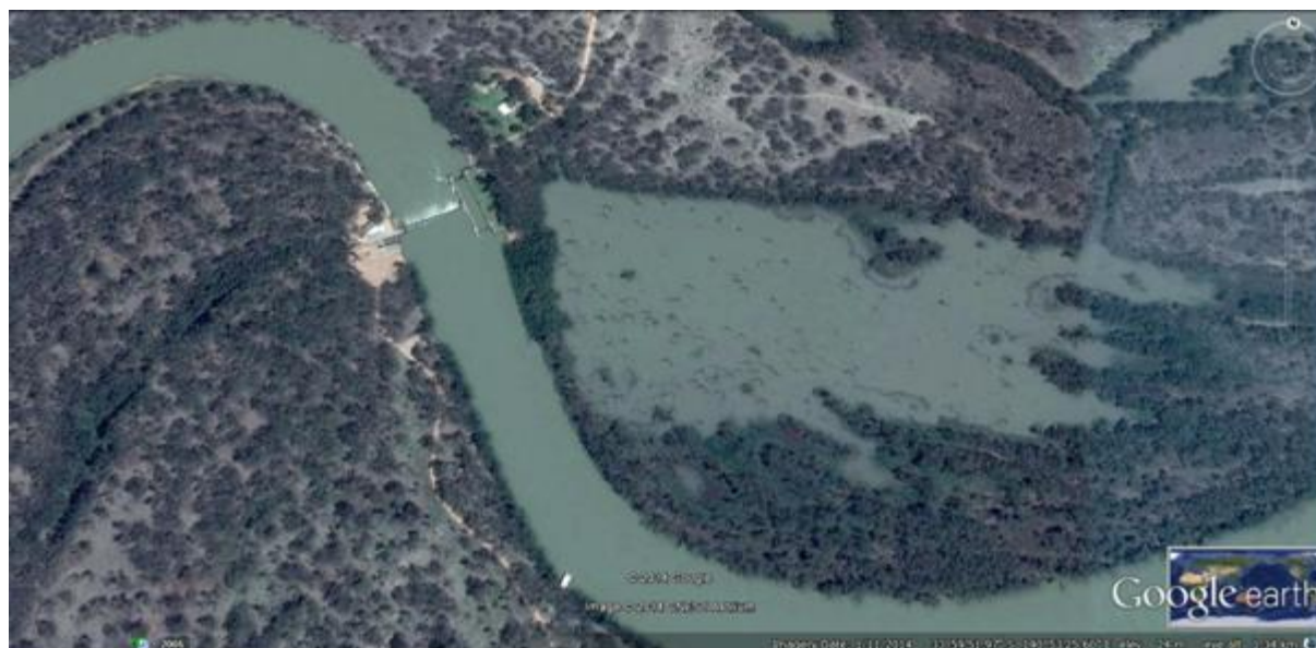
Figure 33. Lock 6 showing the lock on the north (right) bank. The fishway is on the south (left) bank (Source: Google Earth)
