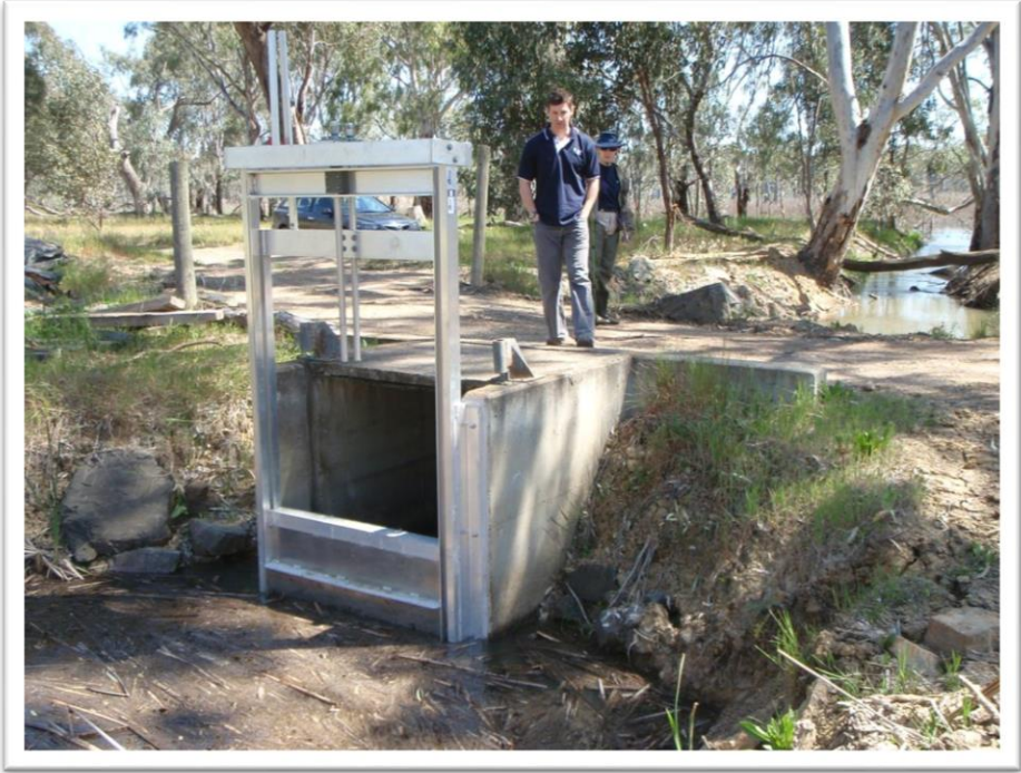
Figure 9: Upgraded inlet structure at Black Swamp 2008
