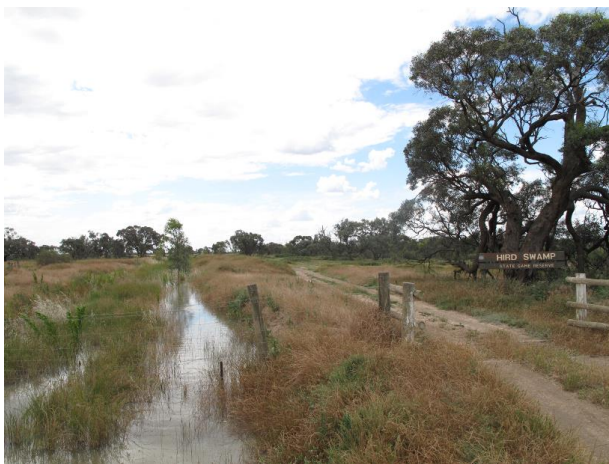
Figure 8: Delivery channel entering Hird Swamp reserve, prior to desilting works being undertaken (October 2010).
