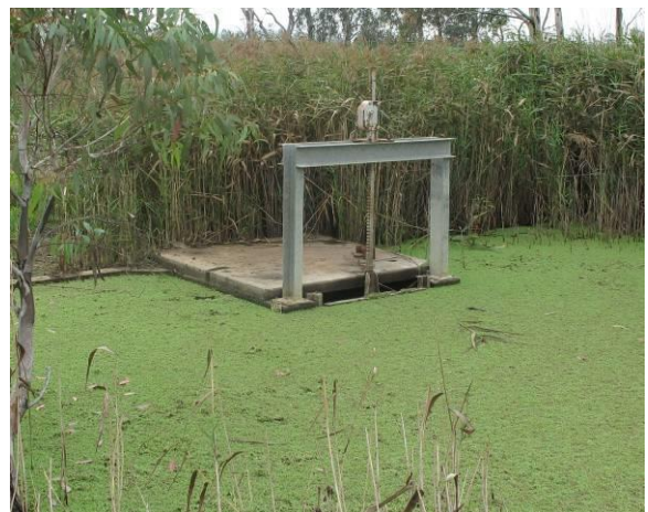
Figure 9: Outlet structure from Hird Swamp west to Pyramid Creek (April 2011).
