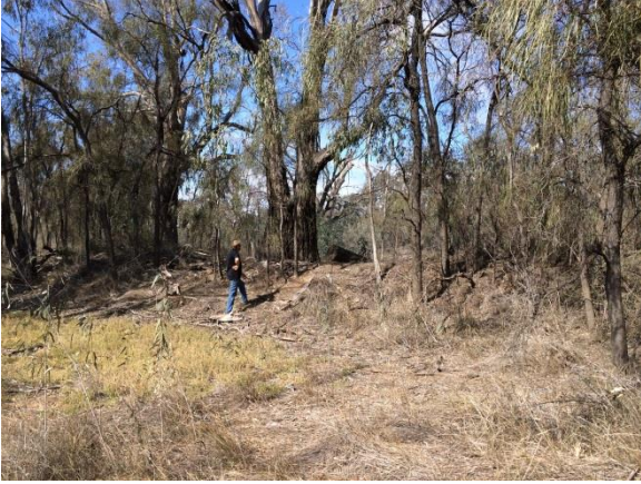
Impediment 5 is a long levee completely crossing the creek bed. A narrow cutting and culvert has been constructed to the east of this levee.
