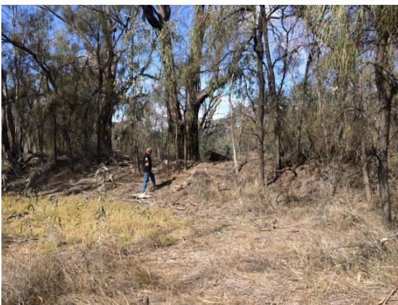
Figure 17 - Levee across Burra Creek at Impediment Site 5
