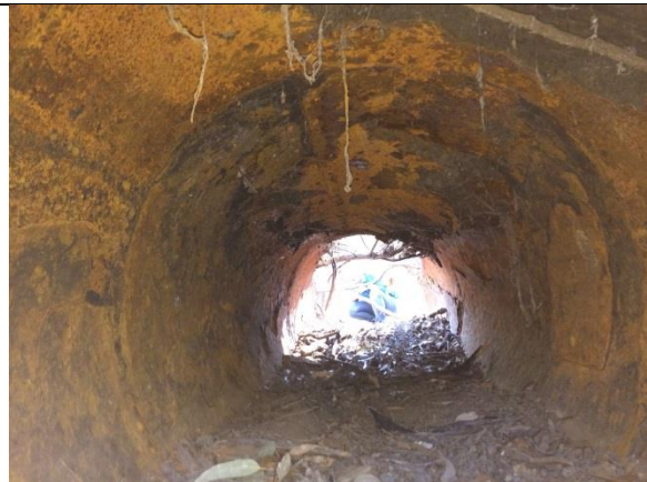
An internal view of the pipe culvert at Impediment 6.
