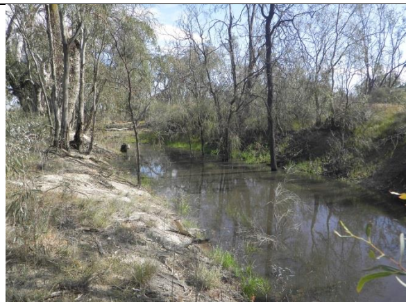
A narrow cutting has been excavated around Impediment 17. The impediment at this location is no longer serves any obvious purpose.
