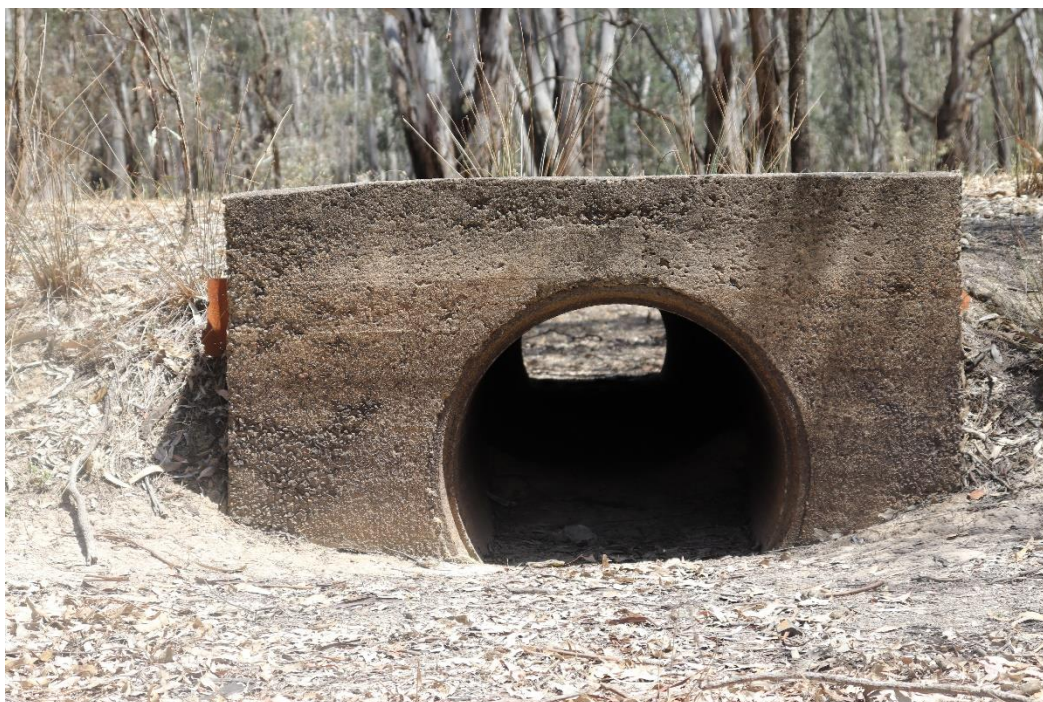
Figure 16: Road culvert acting as a floodrunner constraint.
