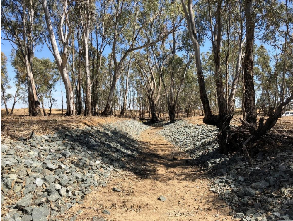
Figure 15: Delivery channel enabling the delivery of water to Loch Garry
