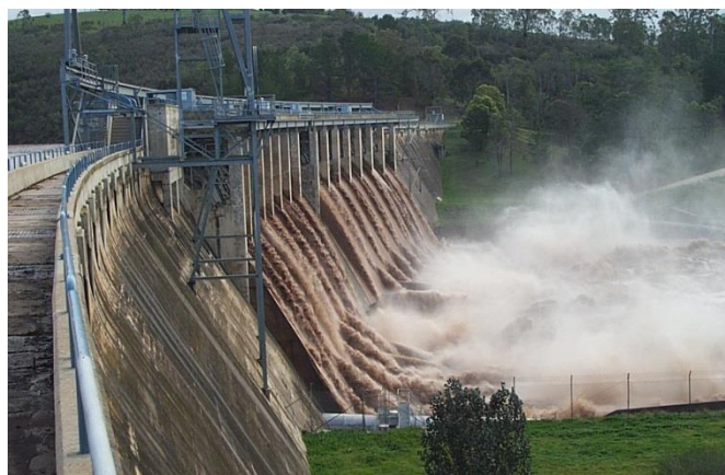
Glenmaggie weir under flood
