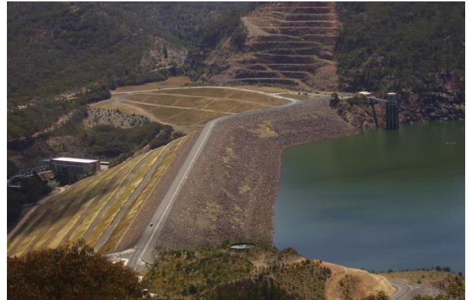
Lake Eildon embankment dam
