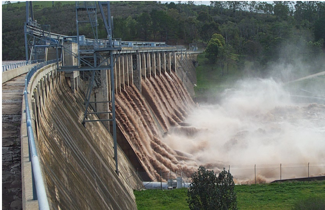
Glenmaggie Weir under flood
