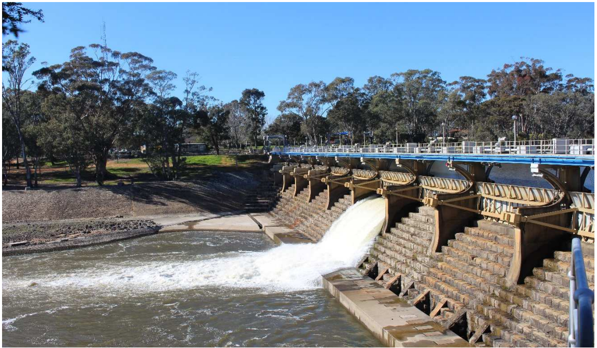
Figure 5 Goulburn Weir (GMW)
