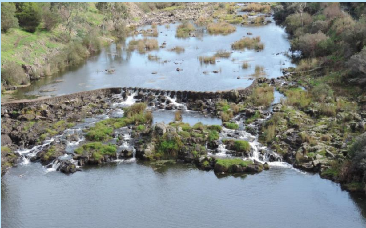
Figure 1: Buckley Falls fish barrier (supplied by CCMA)
