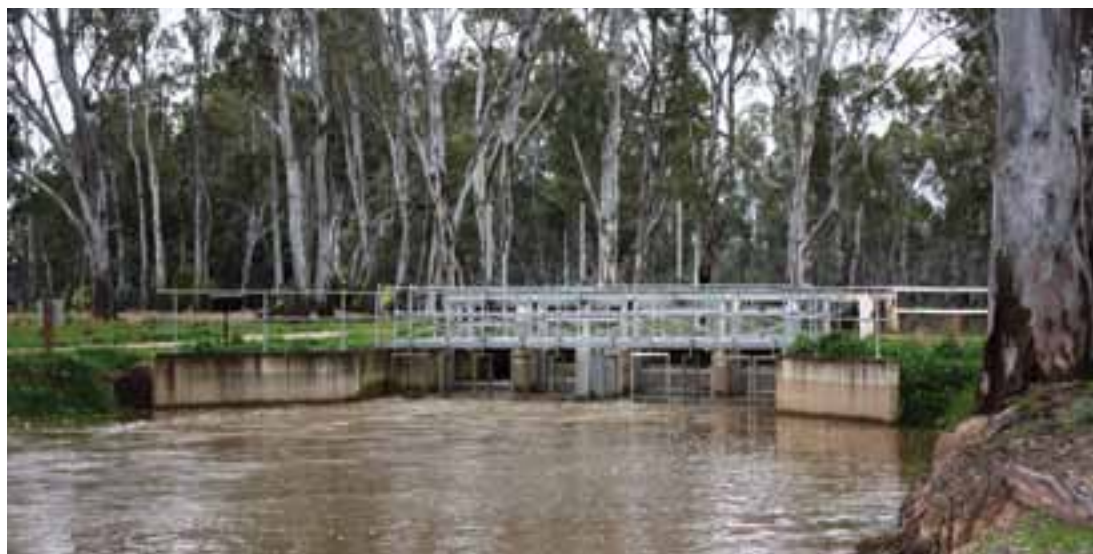
Figure 4.3: Shillinglaws regulator constructed in 2006 on the River Murray (Photo by Melanie Tranter, North Central CMA)
